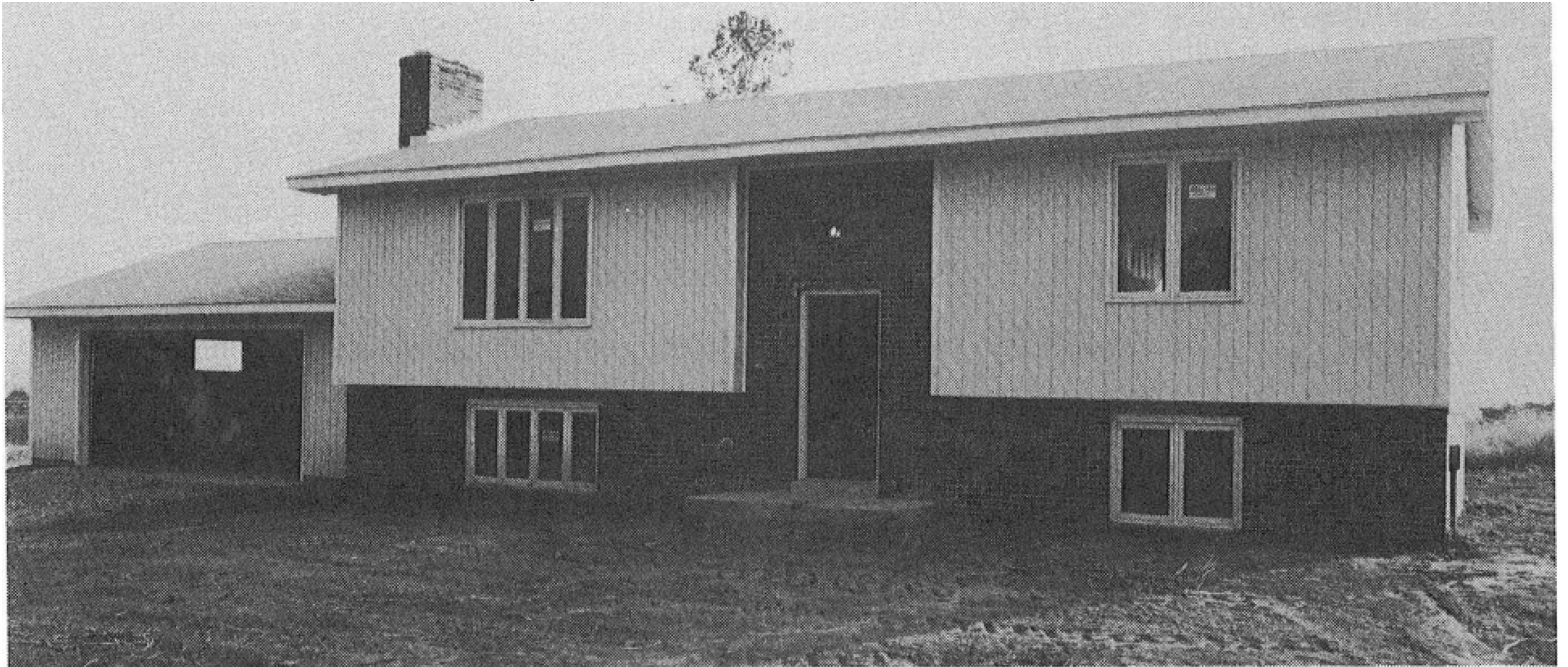
Studies with induced vibrations USBM Test on a wood frame house RI 8896
