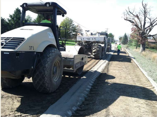
Step 3: Mix cement into gravel with road reclaimer
