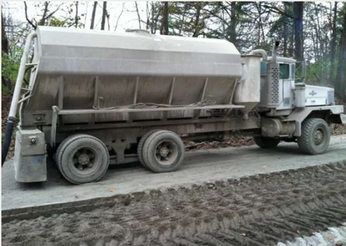
Step 2: Spread cement powder via truck
