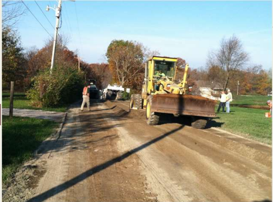
Step 4: Road shaping & compaction
