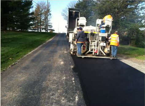
Step 6: Asphalt Paving
