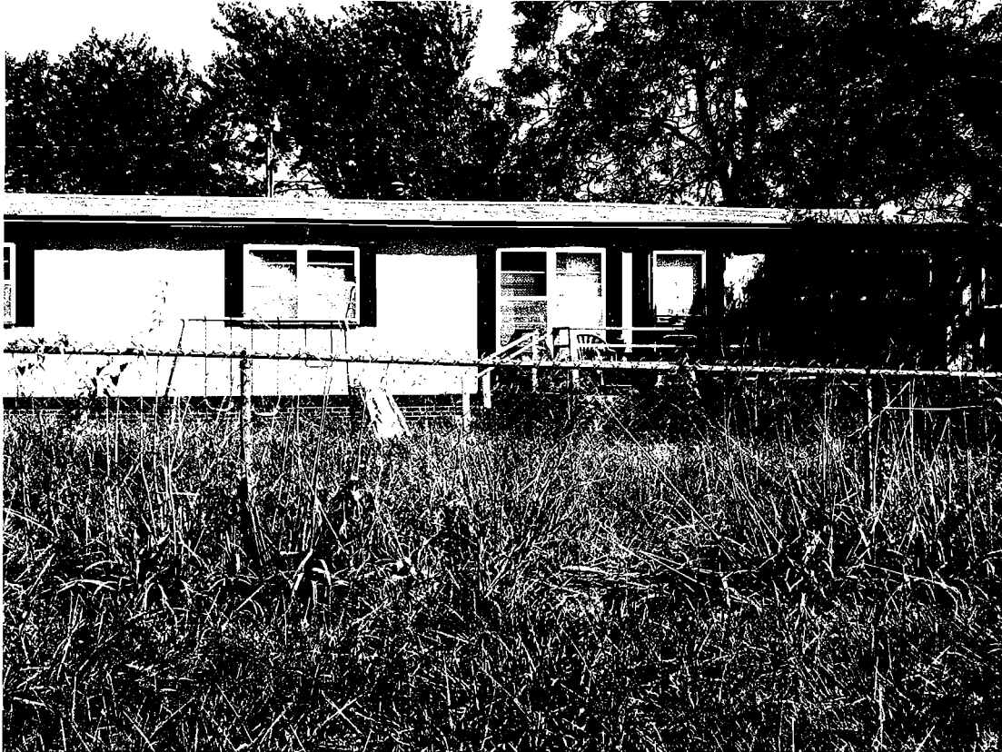
8500 N Wade School Road Pictures taken 8/25/09 by Kala Gunier
