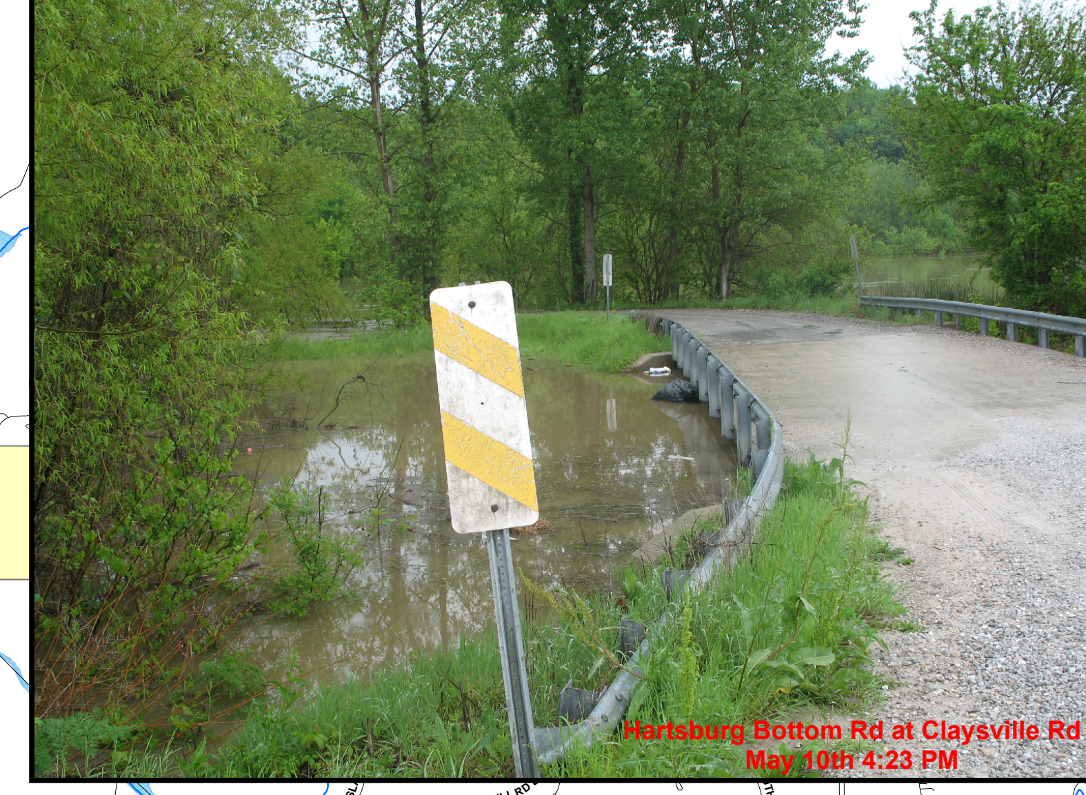
Hartburg Bottom Rd at Claysville Rd May 10th 4:23 PM
