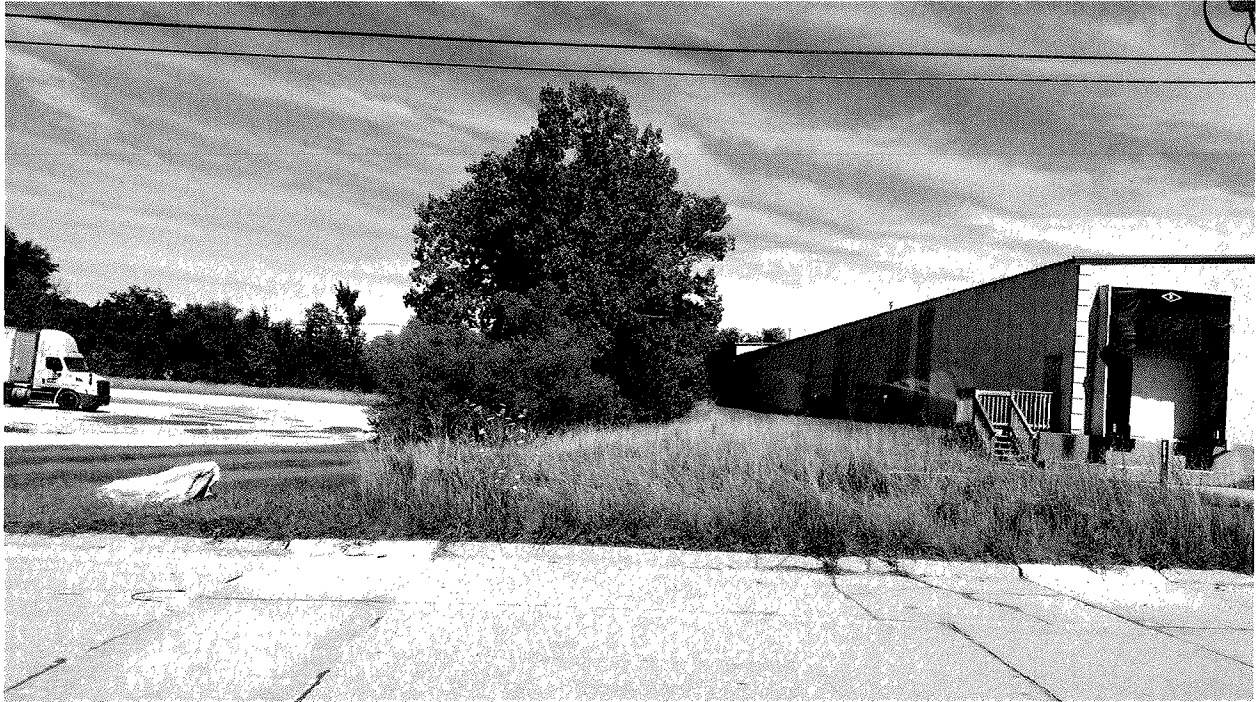
Photographs taken 7/20/15 @ ~ 3:50 pm 4636 N. Interstate Drive
