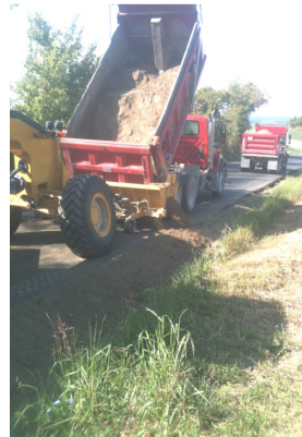
Maintenance crews constructing new shoulders on Claysville Rd.
