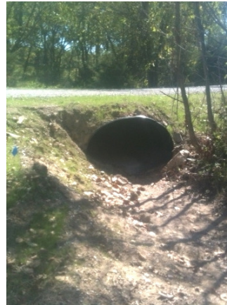
Gilbert Rd - Completed large pipe replacement.
