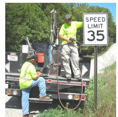
Teresa Shaw and Raenell Mackey installing county signs re-faced with high intensity prismatic background.
