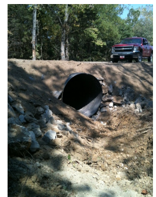
WILLIAMS RD After large pipe installation
