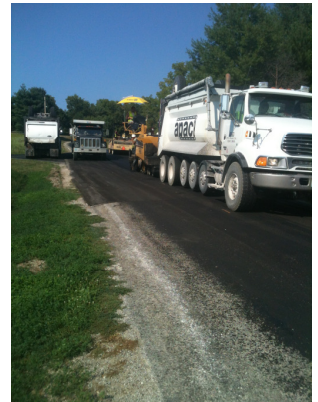
Contractor laying asphalt on Claysville Rd.
