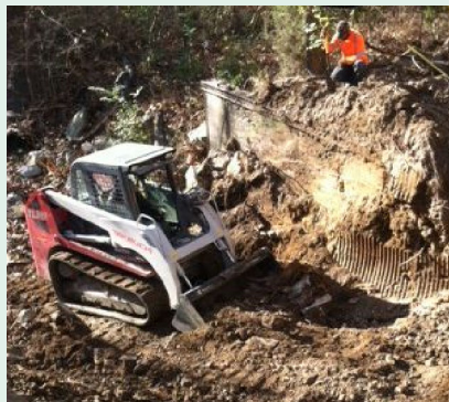
Preparing to bed the culvert pipe on Dusty Rhodes Ln.
