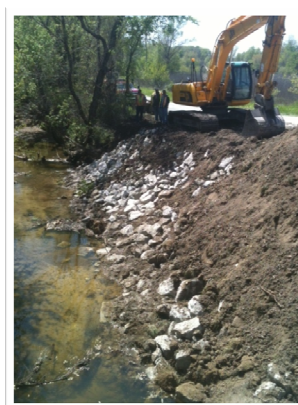
Reusing old concrete to stabilize the creek bank reduced the rock needed to complete the project.
